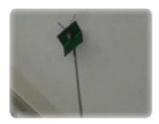
Face the concave side of the installation hooks toward the expansible hooks. Determine the length of the installation hooks from the height of ceiling, then cut off the unnecessary part.
